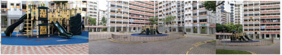
EXISTING PLAYGROUND & HARDSCAPE
